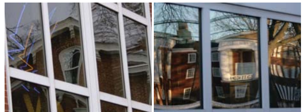
Figure 1. Distortions observed on near-flat window surfaces.
