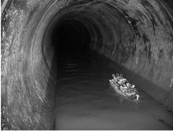
Fig. 1. Spy system in a real sewer with a diameter of 3600mm
