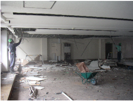
Fig. 2. Current conditions in the works for dismantling offices.
