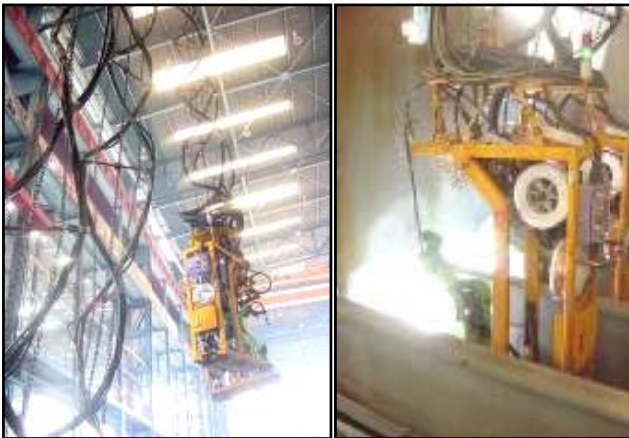
Fig. 3. The use of DANDY for welding in open block
