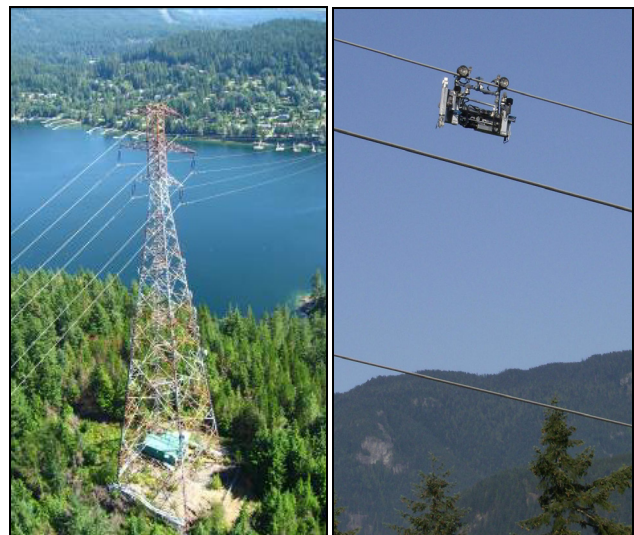
Fig. 1. A mid tower on the 3.0 km crossing, LineScout in action
