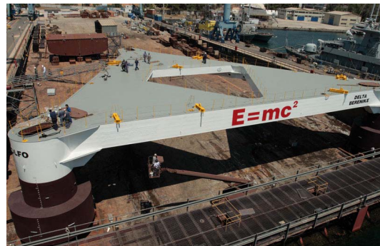
Fig. 1. The triangular floating platform (under construction).
