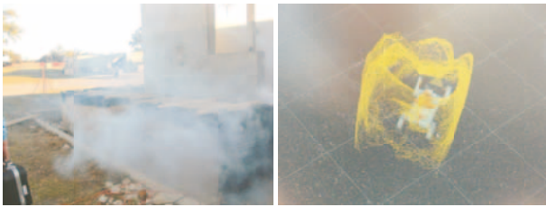
Fig. 12. 3-D scan point cloud measured by TK scanner inside smoke-filled tunnel.
