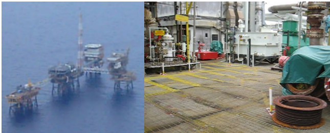
Fig. 7: Offshore platform for real environment testing (aerial view and view of production platform equipped with reflector poles for localization).
