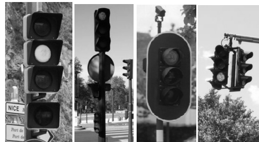
Fig. 1. 1st and 2nd pictures are two French supported traffic lights. 3rd picture is a Belgium supported traffic light. 4th picture is a U.S.A. suspended traffic light.
