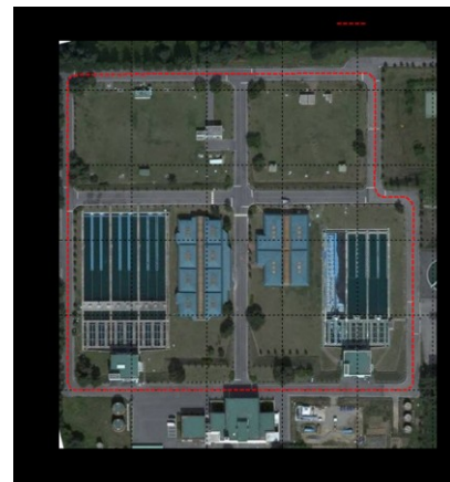
Fig. 6. Asphalt pavement measurements in the Wabu filtration plant.
