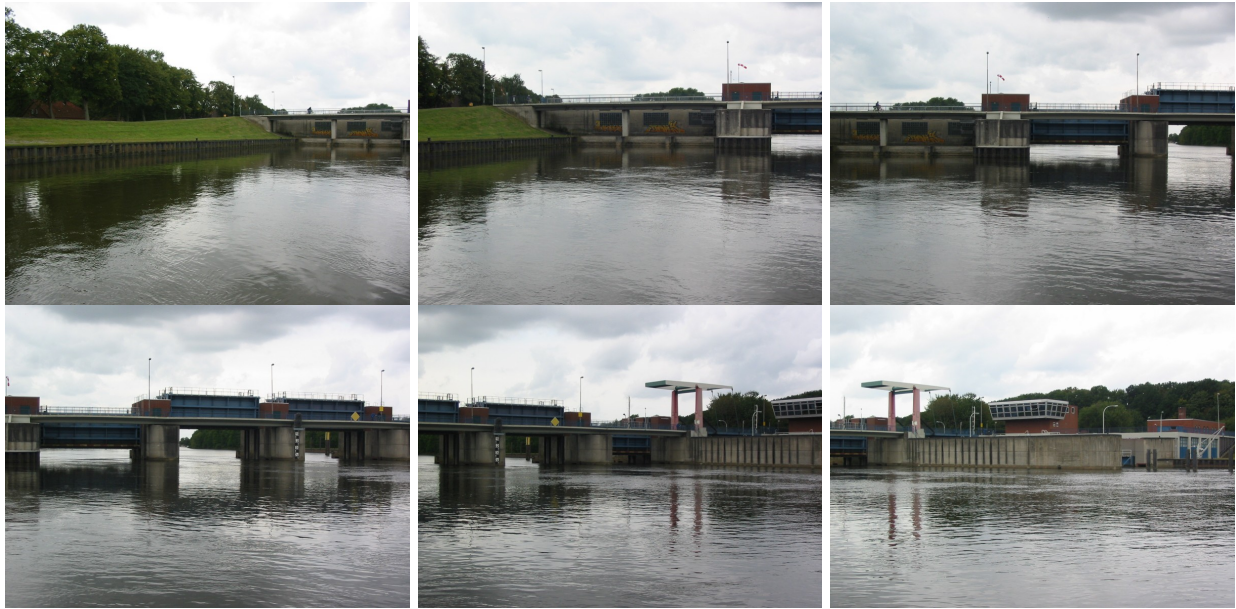
Fig. 1. An overview of the Lesumer Sperrwerk as seen from the river's surface.
