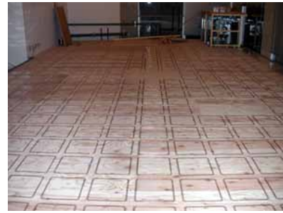
Fig. 1. RFID tags in model room (During Construction).
