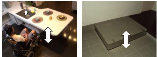
(c) The height of kitchen is automatically adjusted to the height of the wheelchair user. Water supply is also controlled from the server. (d) The elevator for wheelchairs at the entrance works automatically.
