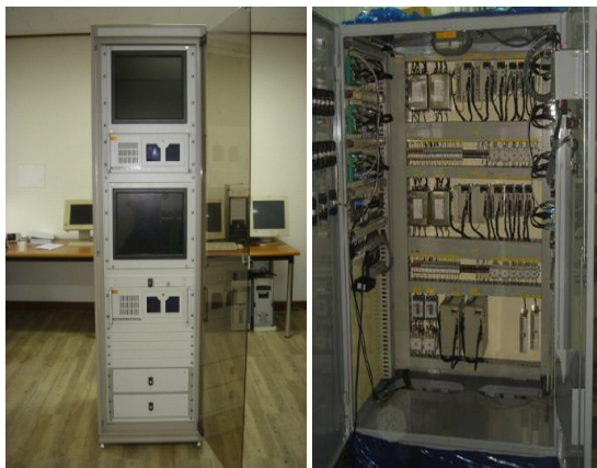
Figure 12: Control system of AUTOMAN.
