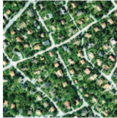
Fig.5 E Single family housing, less “planned” than D
