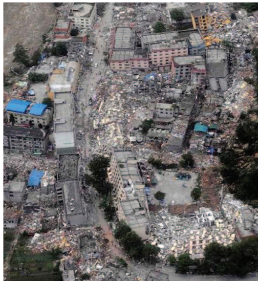
Figure 1. Collapsed buildings in 5.12 Wenchuan Earthquake (Ms 8.1)
